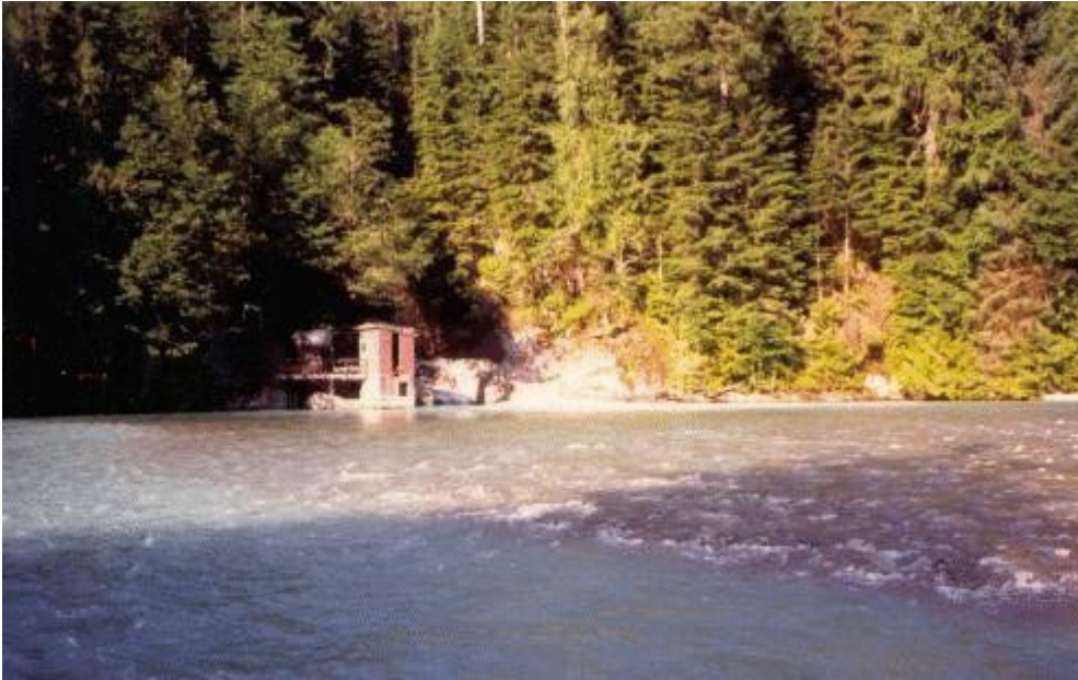
Photograph of the Federal Fish Hatchery on Corbold Creek near Alvin. After traveling through a subterranean channel Corbold Creek boils to the surface just to the right of the small observation building in the background.
