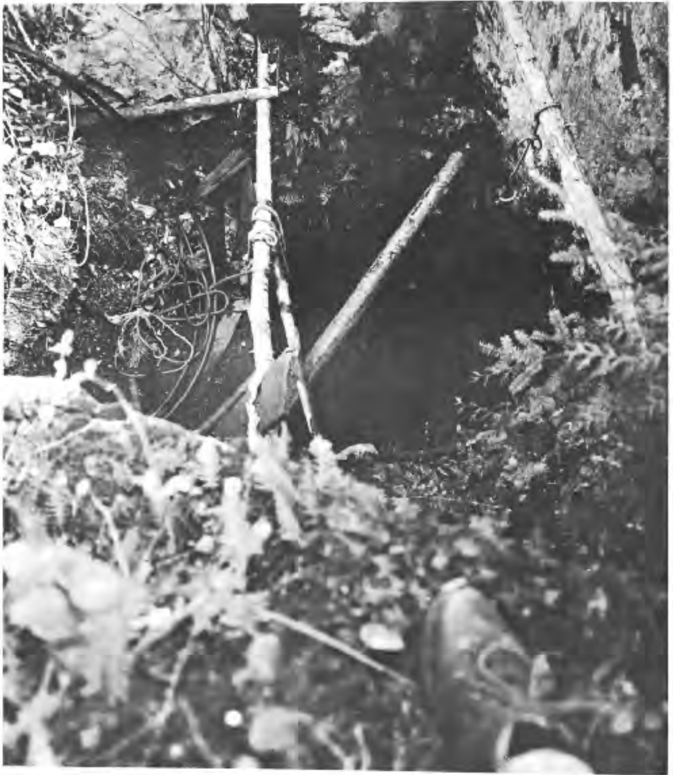
SCOOCH'S MINE ON SHERIDAN HILL. THIS ABANDONED 60 FOOT MINE SHAFT WAS NOT RECORDED WITH THE B.C. DEPARTMENT OF MINES UNTIL LAST YEAR WHEN DANNY SCOOCH STAKED BOTH MINERAL AND PLACER CLAIMS FOR THE ENTIRE VICINITY.
